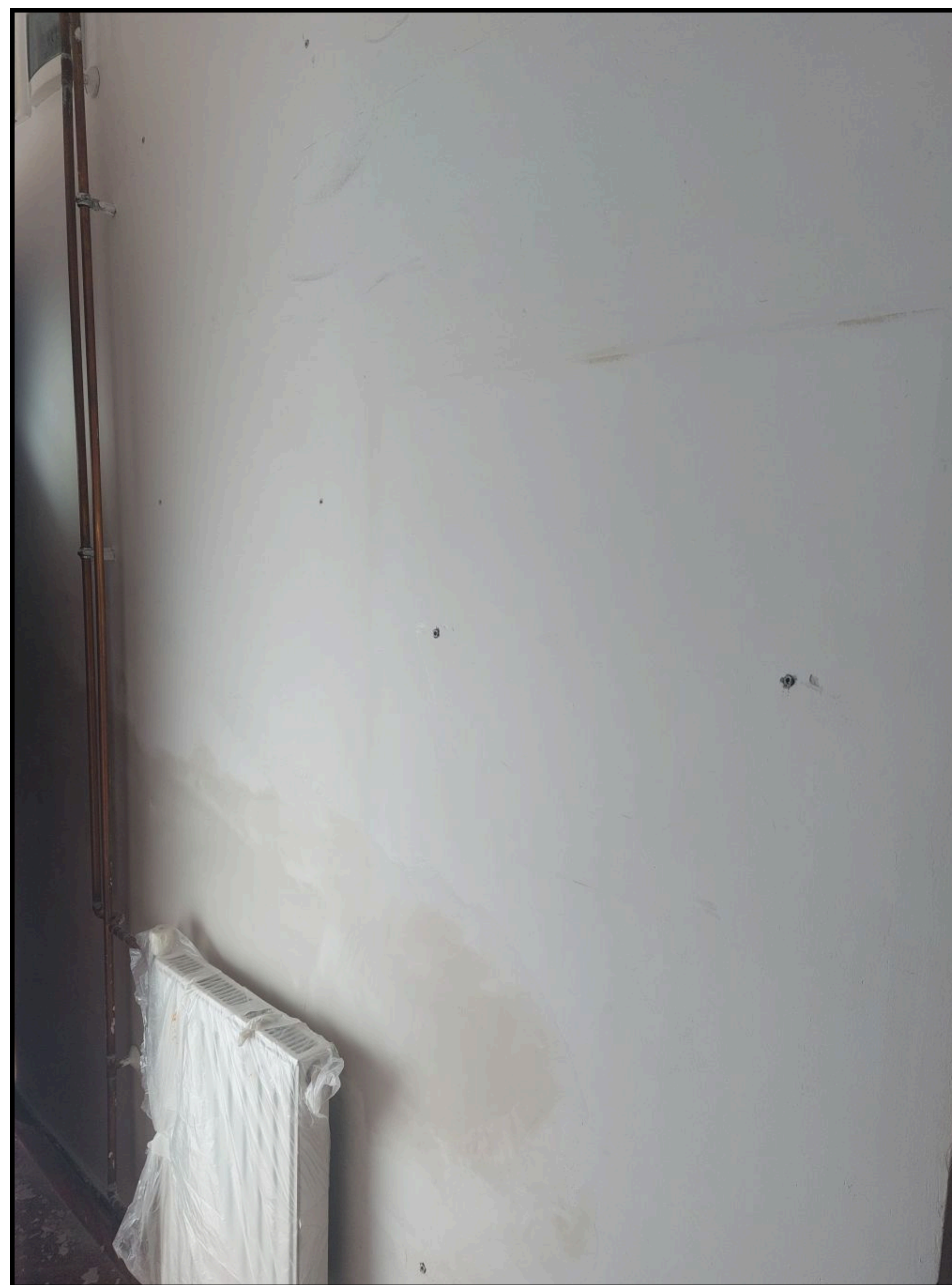
Picture 3: The water-damaged wall after sanding and plastering
